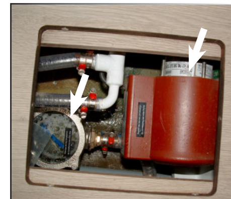
FILTER + SEEWASSERPUMPE
